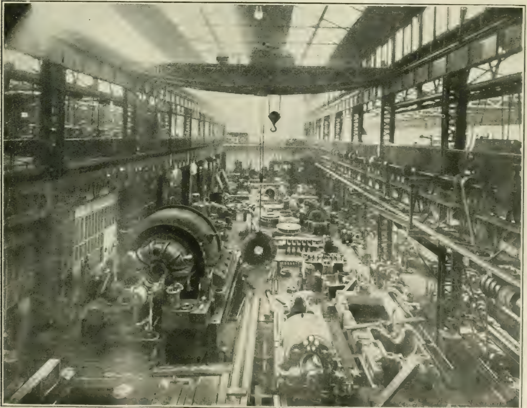
ERECTING BAY OF MACHINE SHOP, FRASER & CHALMERS ENGINEERING WORKS, AT ERITH.
